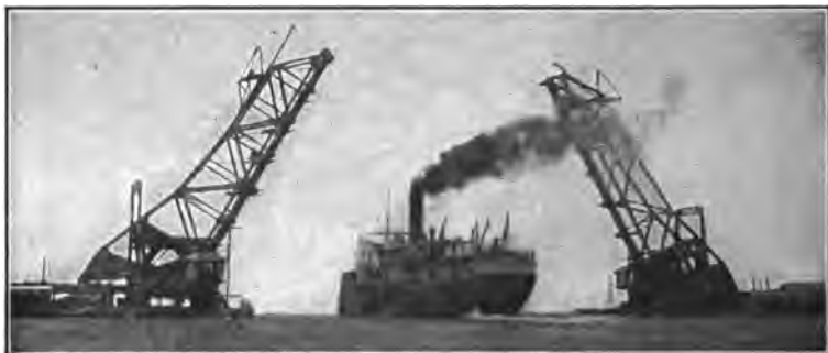
FIG. 262.—Viaduct between India and Ceylon, built entirely by native labor under white supervision. (Scherzer Bridge Co., Chicago) (See Fig. 261.)
